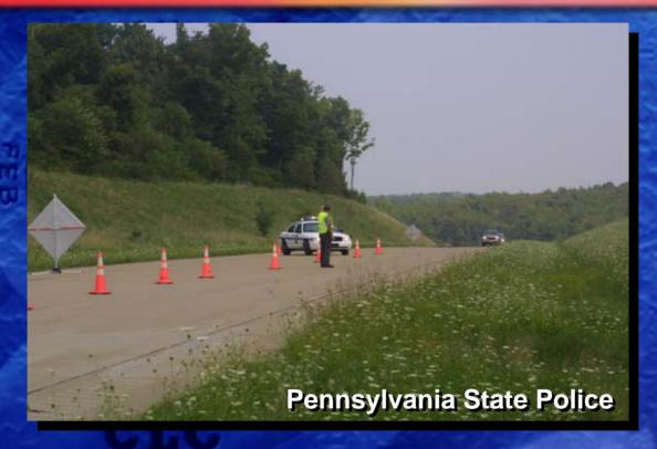
Is safer to divert traffic with advanced placement of signs and cones rather than relying on warning lights and vehicles.
